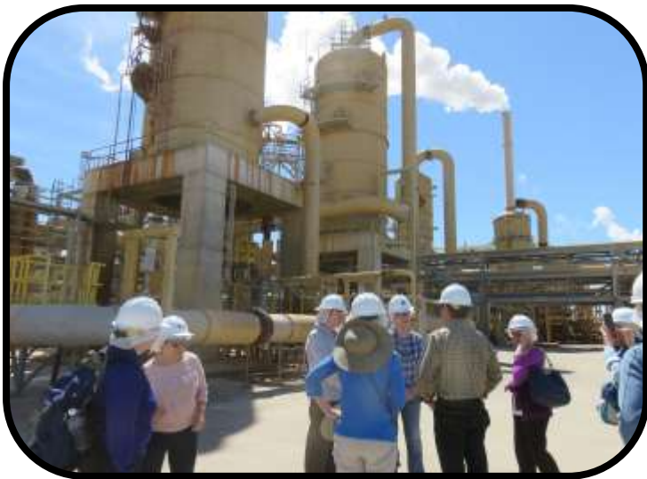
Figure 1 Hudson Geothermal Plant
